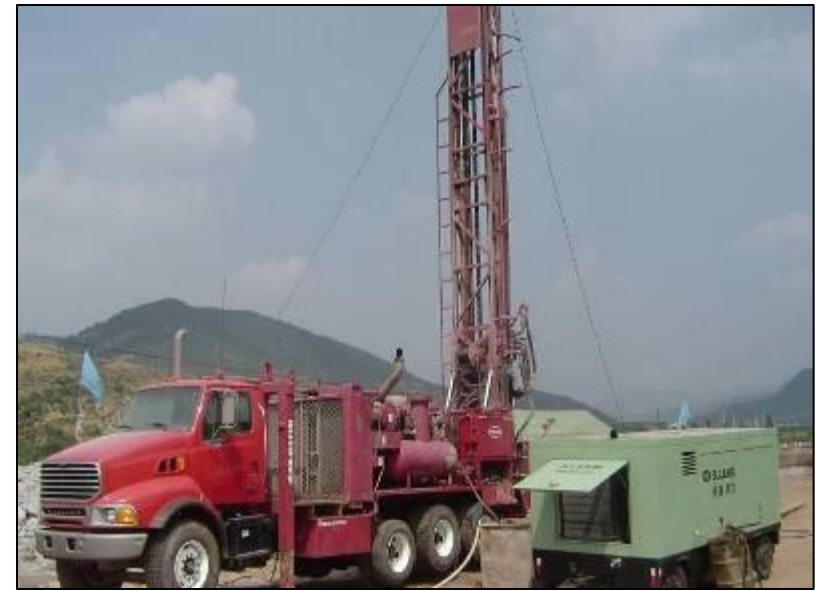
Mobile drilling rig
